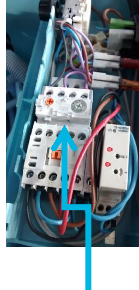
Non modular units: disconnect red cable or use cleaning switch If available.
